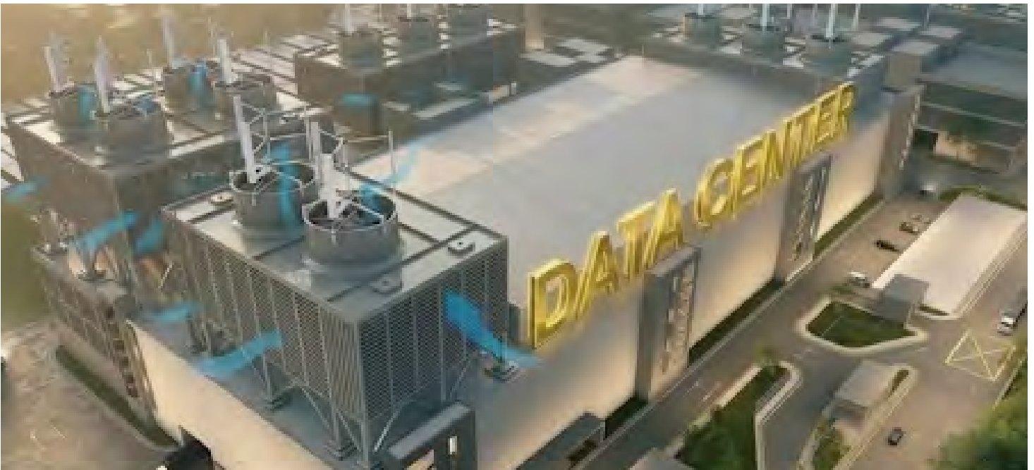
Artist's impression of the Cross-Axis Wind Turbine (CAWT) integrated into a data center cooling system.
